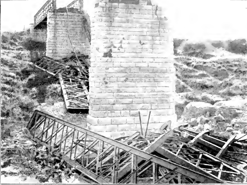
ANOTHER VIEW OF THE DESTROYED BRIDGE OVER THE VET RIVER.
